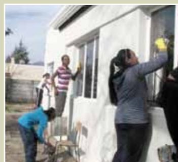
Learners hard at work on the windows
